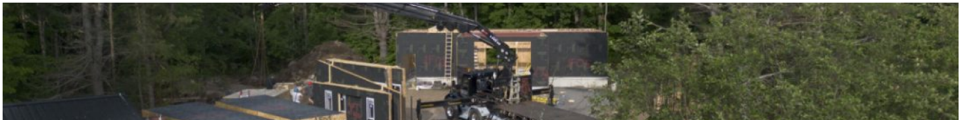
DAY 01 CRANE-ASSISTED SET · PANELIZED ENVELOPE ARRIVING ON A RURAL LOT
